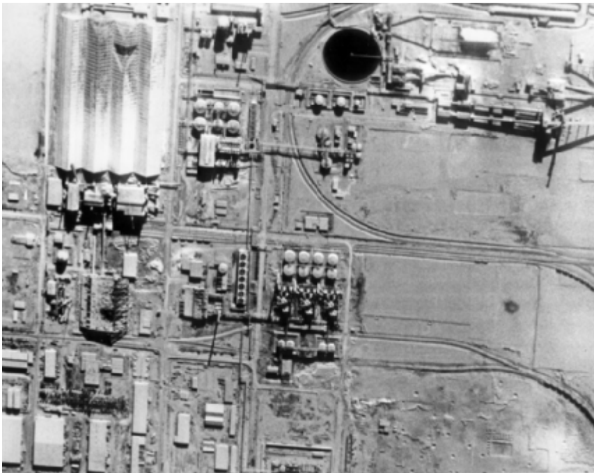
An F-14A Tomcat from Fighter Squadron 32 took this photograph of bomb damage at an Iraqi fertilizer plant, using the tactical air reconnaissance pod system, or TARPS.
