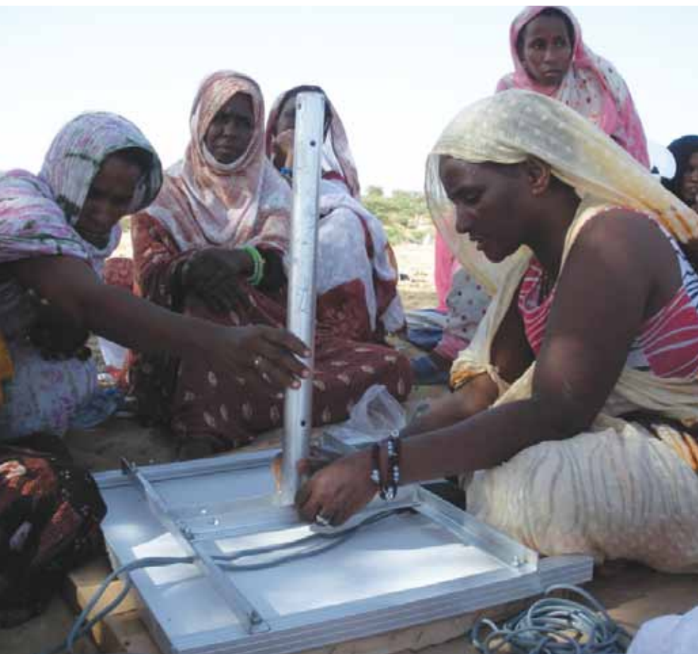
These Mauritanian women install solar panels in their village after training at Barefoot College in India, where they learned to be solar engineers. They receive income for their work.
