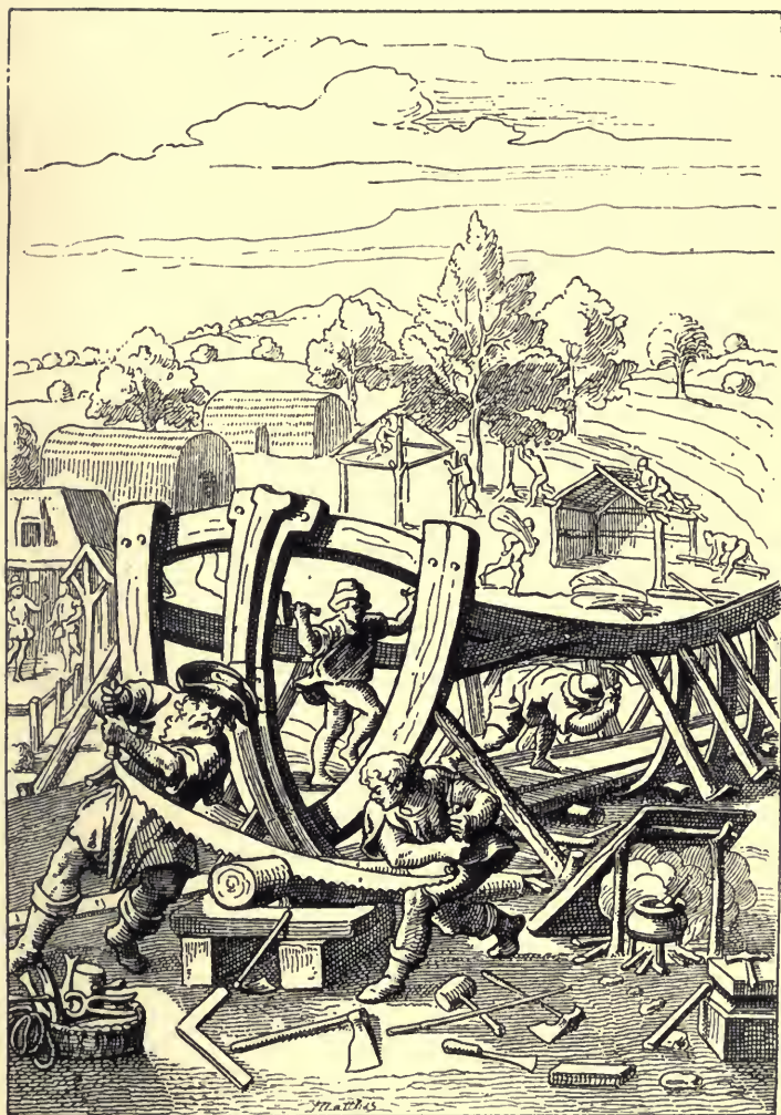
Building a caravel.
