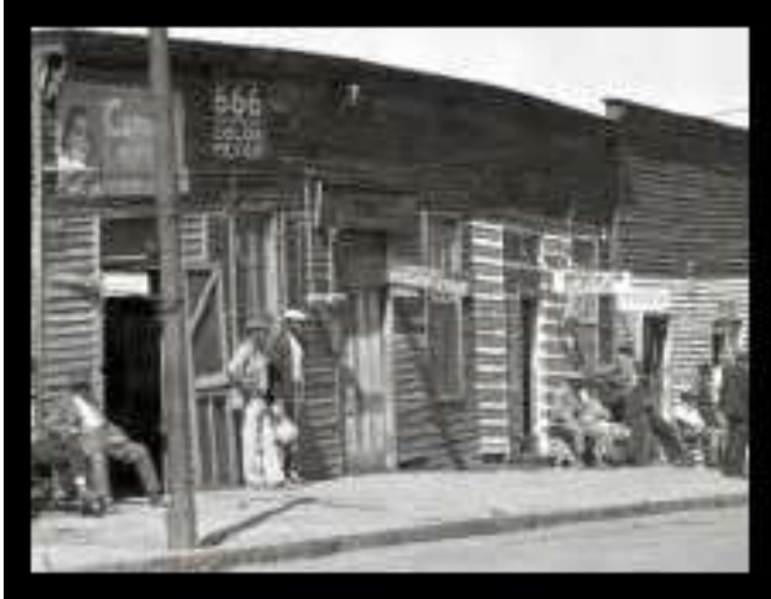
Shops along Left-over Main. Hyannis, 1935
