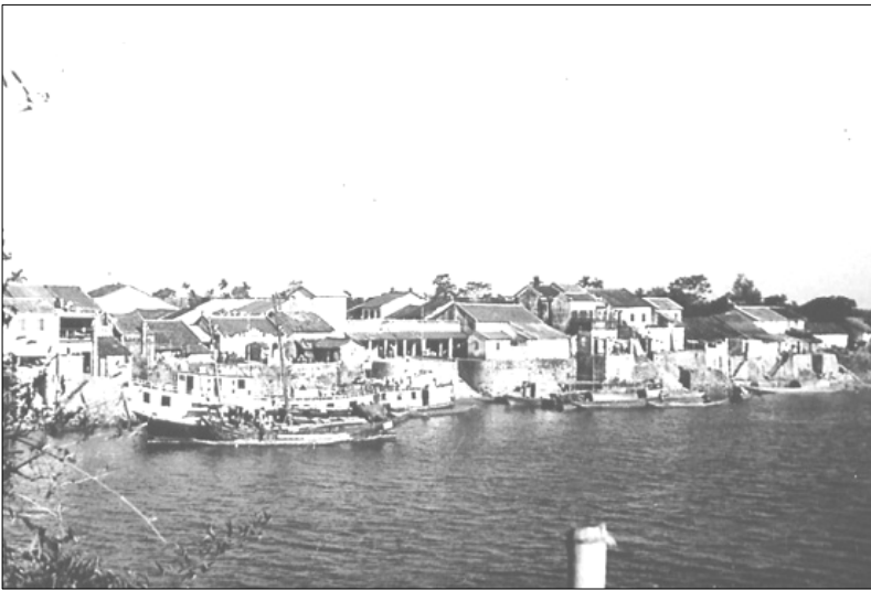
The Goc Khe Pier, Moncay (Photo BB)
