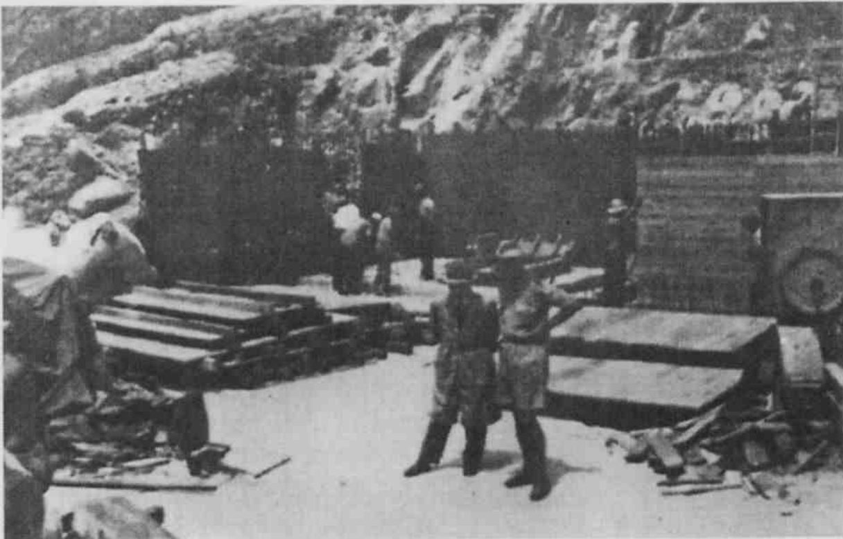
Gun emplacements under construction on Tomaree Head about 1941. Timber formwork is being positioned prior to pouring concrete.
