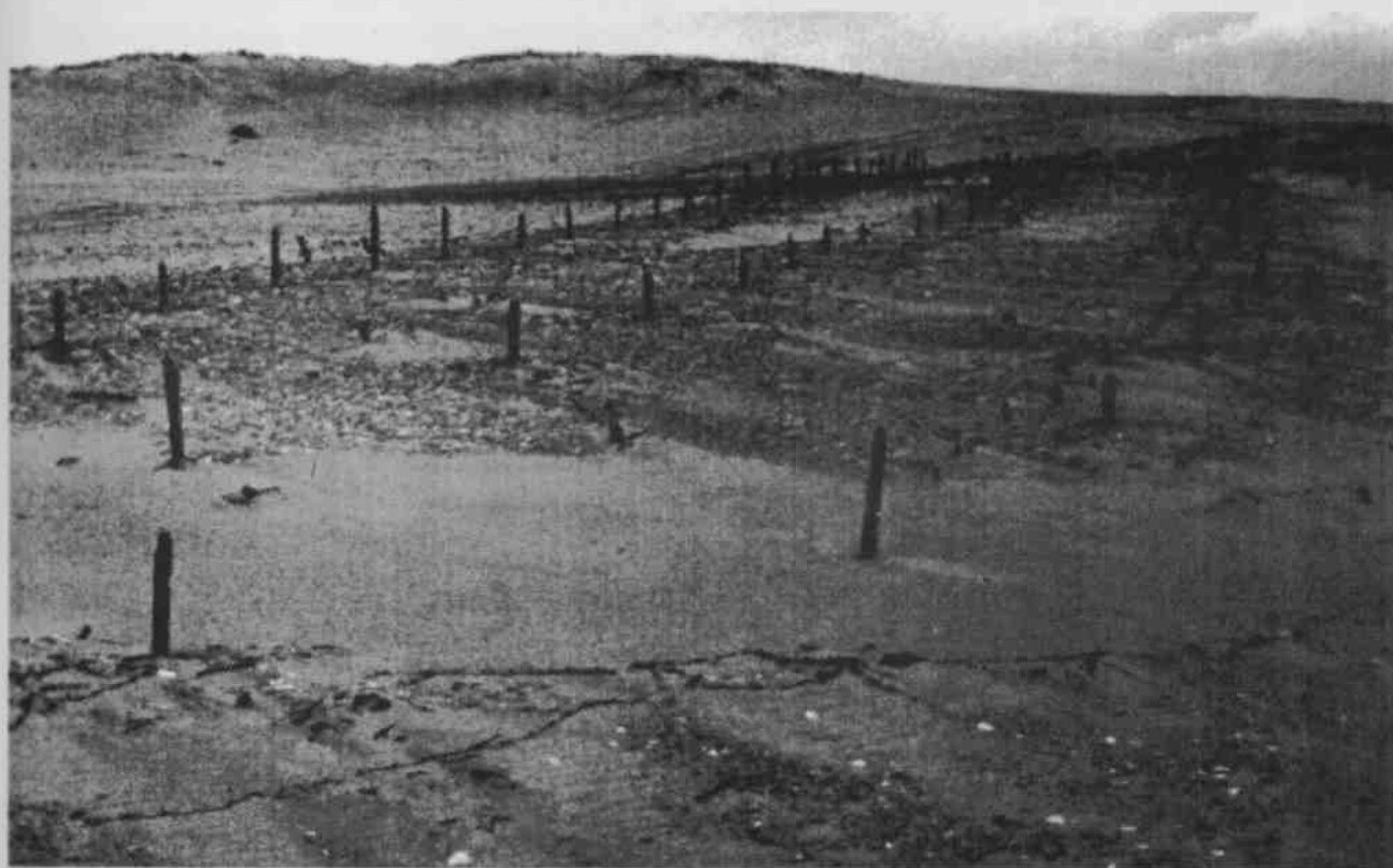
This photograph taken in 1998 shows the remains of the barbed wire entanglements on Stockton Beach. Here 3 rows of star pickets supported coils of barbed wire. Similar methods were probably used on Zenith Beach.
