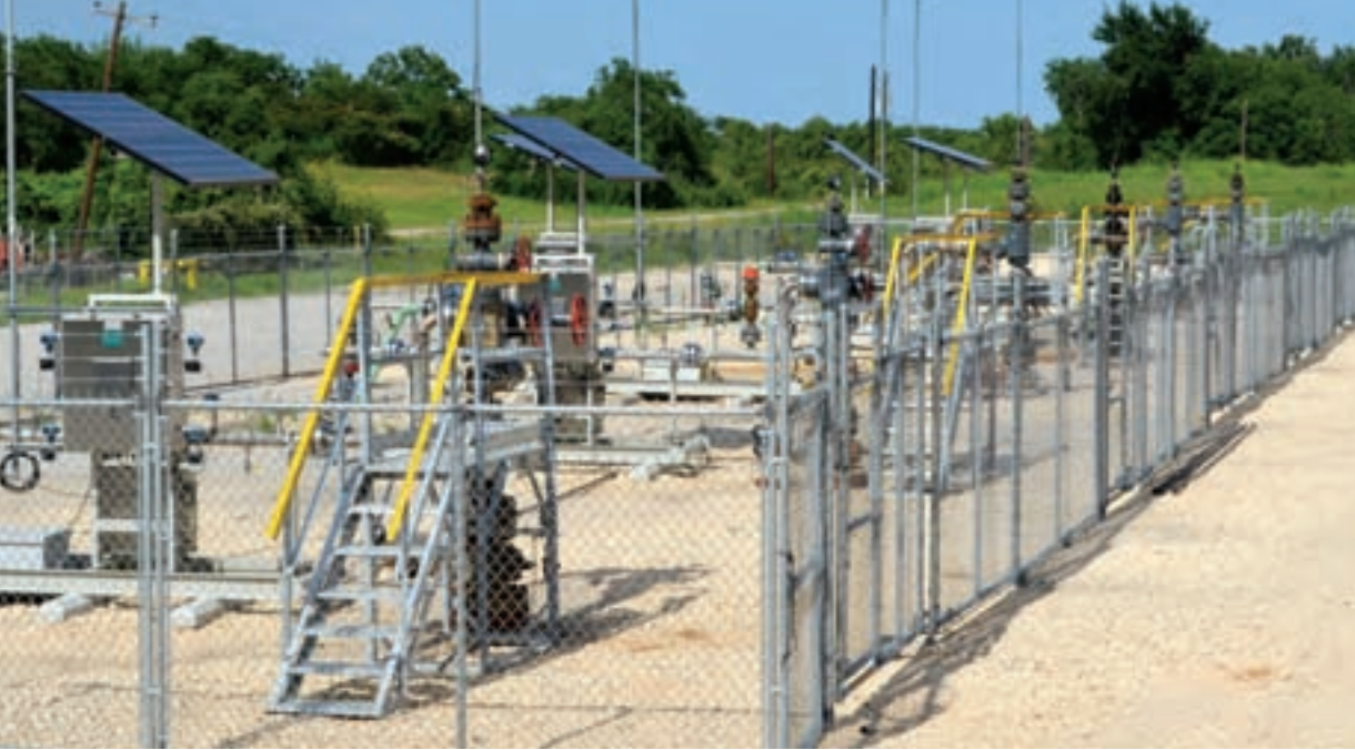
Above: Solar powered well metering and telemetry system, Hastings Field in Alvin, Texas.
