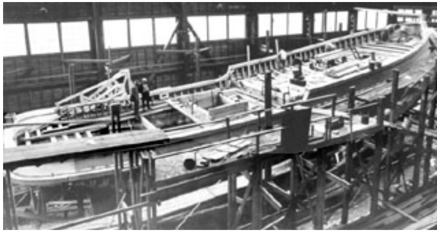
Building the John N. Cobb, NOAA
