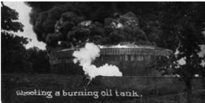
Bottom, right: This gun was used to shoot oil tanks when they caught on fire. The shot was often a 3" ball that would leave a hole in the side of the tank so the oil could drain into a dyke that surrounded the tank.
