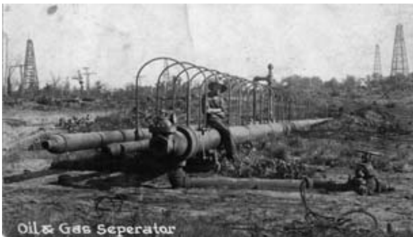
Left: An early photograph of an innovative oil and gas separator in the 1910s.
