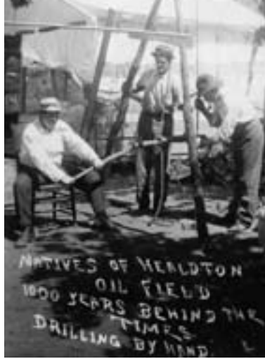
Top: Drilling an oil well by hand.
