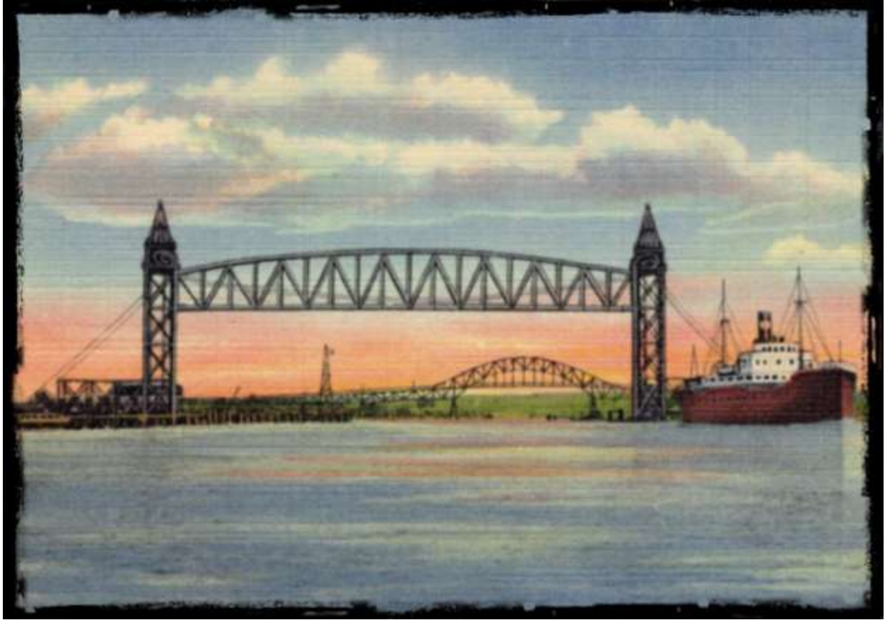
The Cape Cod Canal Railroad Bridge.
