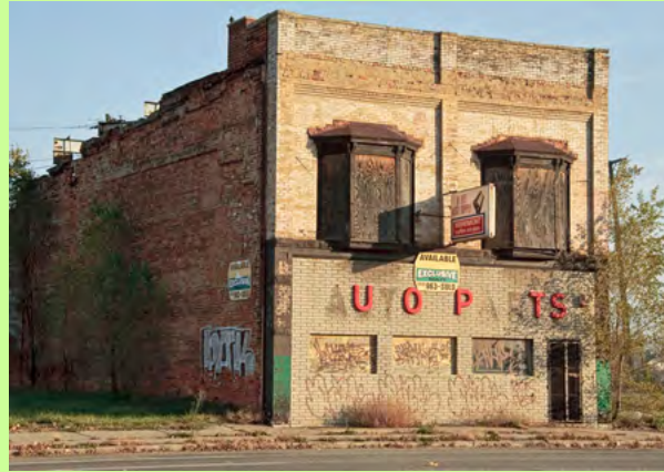
Figure 10.2 This dilapidated auto supply store in Detroit is a victim of auto industry outsourcing. (Photo courtesy of Bob Jagendorf/flickr)
