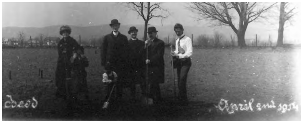
❖ The groundbreaking for the expansion of Hood College in April 1914.
