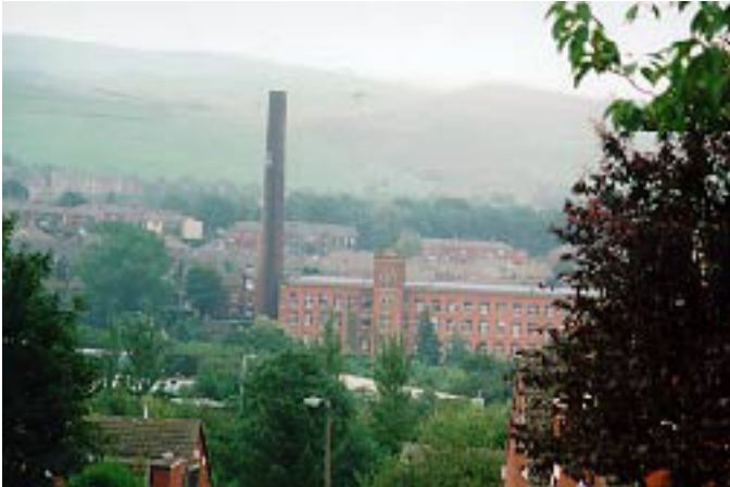
Photo 11 Typical Mill at Oldham
