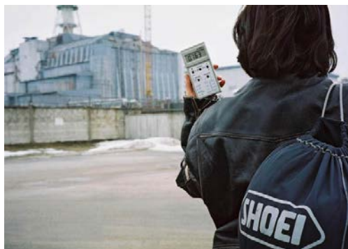
Figure 31.23 The Chernobyl reactor. More than 100 people died soon after its meltdown, and there will be thousands of deaths from radiation-induced cancer in the future. While the accident was due to a series of human errors, the cleanup efforts were heroic. Most of the immediate fatalities were firefighters and reactor personnel. (credit: Elena Filatova)
