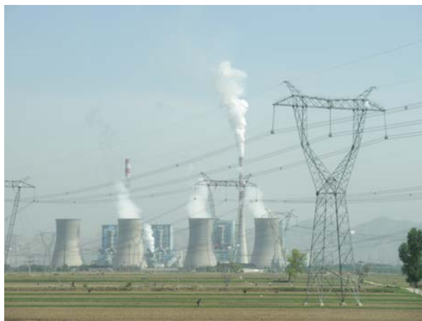
Figure 7.25 Tremendous amounts of electric power are generated by coal-fired power plants such as this one in China, but an even larger amount of power goes into heat transfer to the surroundings. The large cooling towers here are needed to transfer heat as rapidly as it is produced. The transfer of heat is not unique to coal plants but is an unavoidable consequence of generating electric power from any fuel—nuclear, coal, oil, natural gas, or the like. (credit: Kleinolive, Wikimedia Commons)
