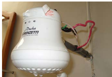
Figure 20.41 On-demand electric hot water heater. Heat is supplied to water only when needed. (credit: aviddavid, Flickr)
