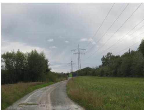
Figure 24.10 This high-voltage traction power line running to Eutingen Railway Substation in Germany radiates electromagnetic waves with very long wavelengths. (credit: Zonk43, Wikimedia Commons)
