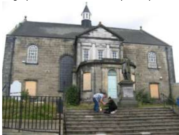
St Andrews Erskine Church as a building at risk
