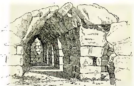
FIG. 74. GALLERY IN THE SOUTH WALL AT TIRYNS
