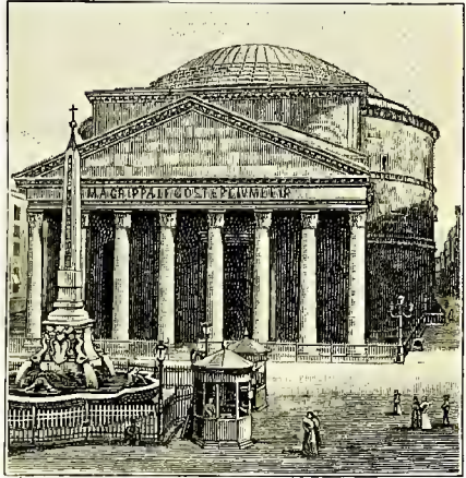
FIG. 188. THE PANTHEON, AT ROME (Present condition)
