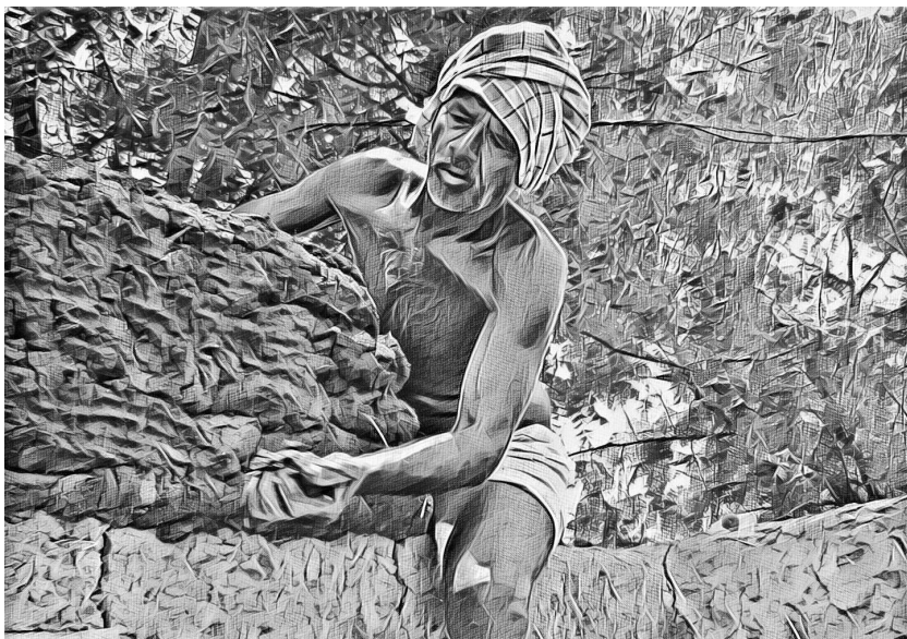
Yellaiah immersed in the construction of mud wall of my house
