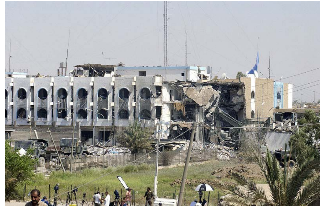
Figure 6.17 Physical damage to an asset can result in an impairment loss.
