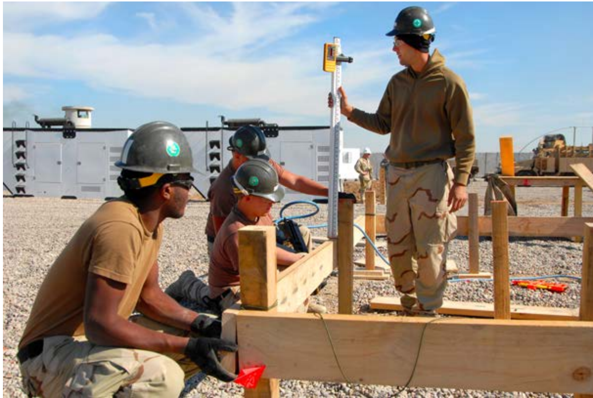
Figure 1.6 Laying a Foundation for Building
